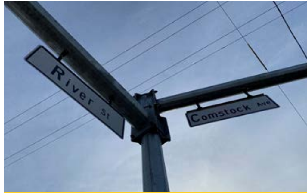
New signal mast arms at the intersection of River Street and Comstock Avenue.
