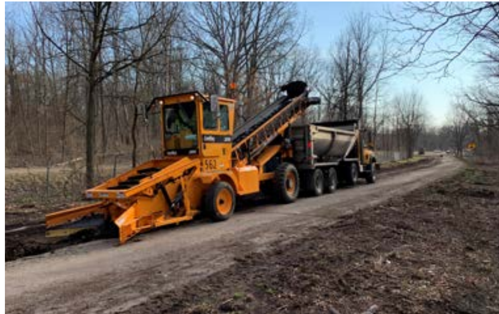
High shoulder removal work in Charleston Township.
