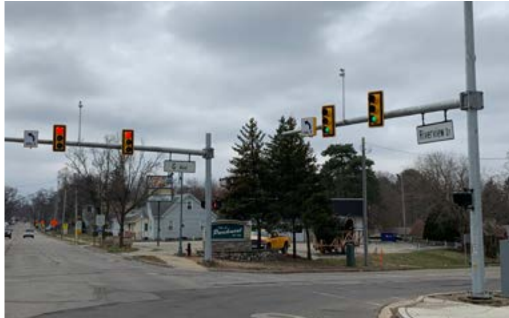
Signal upgrades at G Avenue and Riverview Drive.
