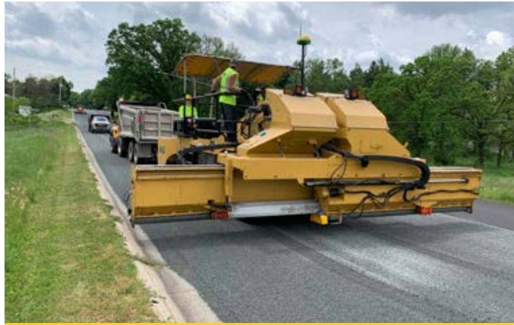
Chip sealing on 34th and M-89.
