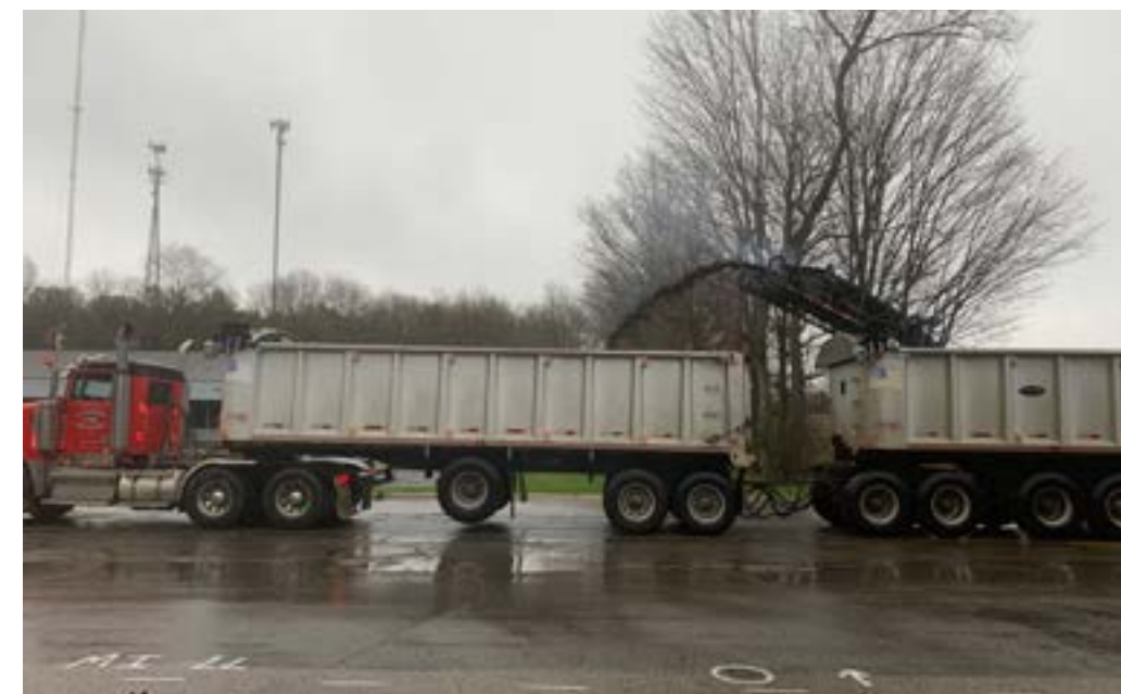
Milling 34th Street.
