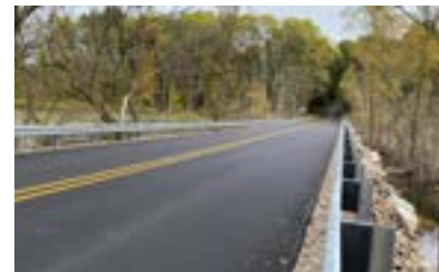
8th Street - one of the flood repairs in 2020.
