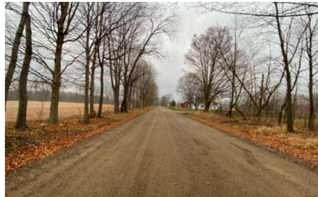
YZ Avenue east of 46th Street after pulverization.
