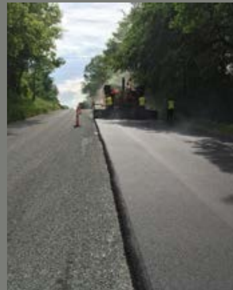
HMA overlay on a Texas Underseal
