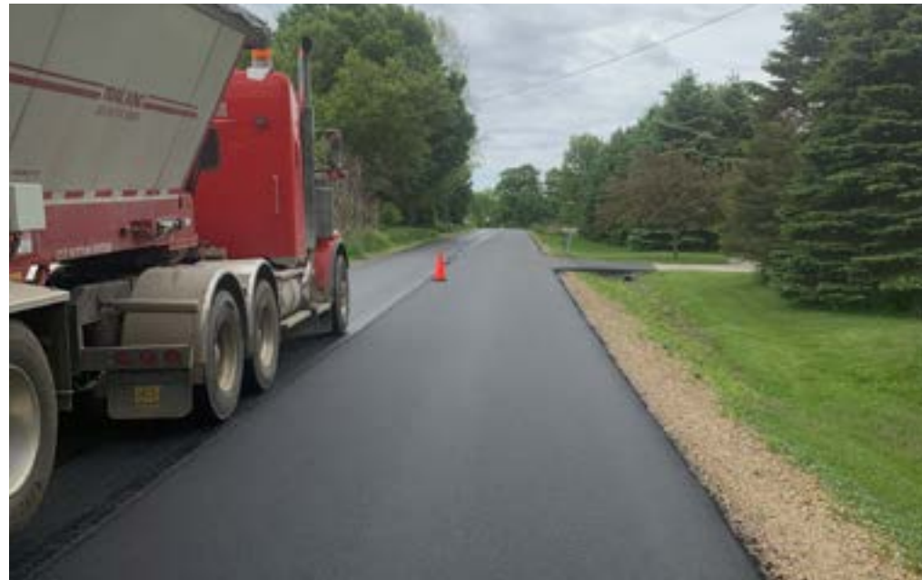
HMA Overlay on 39th Street between V Avenue and U Avenue.
