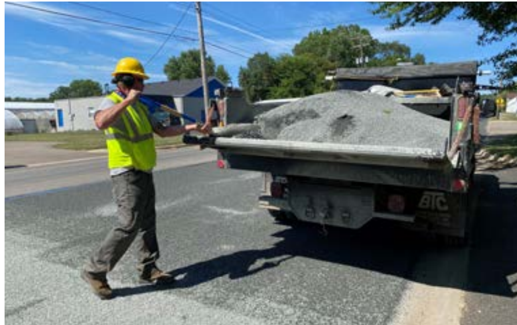
Chip seal on Mosel Avenue between Westnedge Avenue and Riverview Drive.
